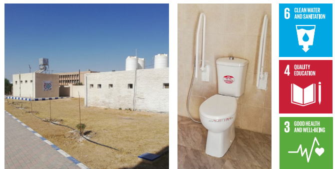
Sanitary facilities constructed by Sanitation for Millions
