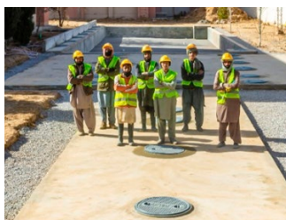
The main structure of new toilets and handwashing facility is ready
