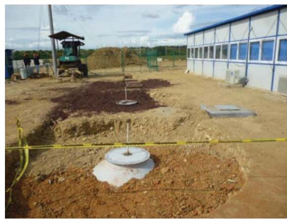
Figure 4: Using prefabricated fiber-reinforced plastic or monolithic concrete (around 500 people for this office building in Miramar) the installation time can be reduced to 3 days.
