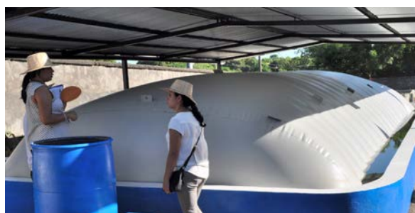
Figure 5: Anaerobic baffled reactor (T.3) with membrane cover
