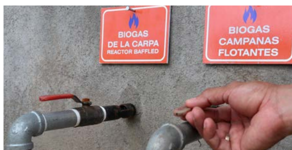
Figure 4: Biogas outlet from ABR (left) and Biogas reactor (right)
