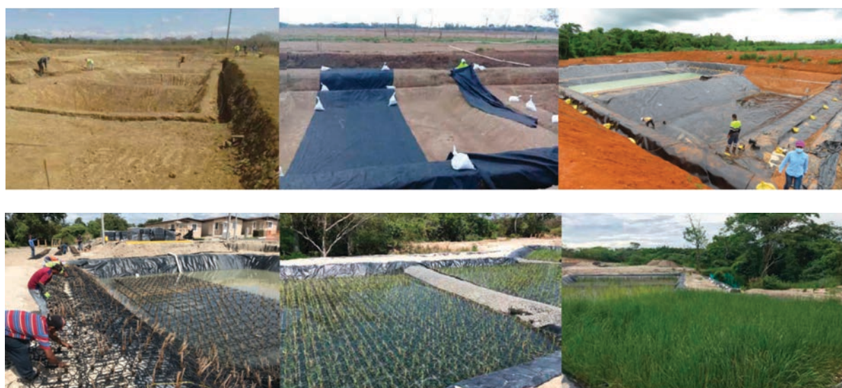
Figure 4: Overview of the individual construction steps. Earthworks, laying of the geotextile, installation of the watertight geomembrane as well as planting of macrophytes, commissioning and fully operational floating treatment wetland.
