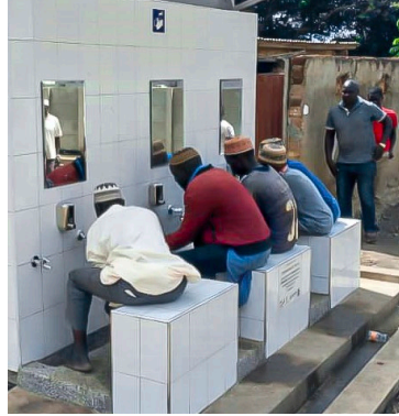
Worshippers at a mosque using the new ablution station
