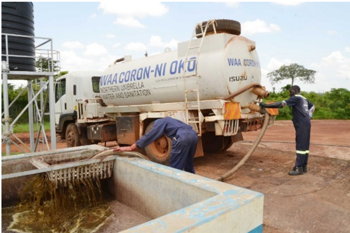
Figure 3: Private operator during the sludge disposal at the FSTP at Aminteng, Apac Municipality.
